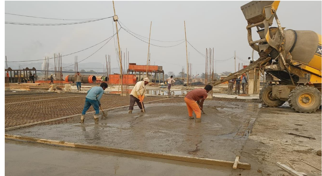
Waste Management Plant construction at Guwahati
